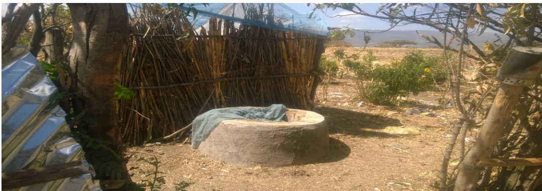
Plate 4: The inlet filled with dry dung which covered with dress.
