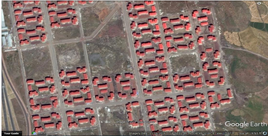
Figure 3-3 : Building and Roof orientation assessment using Google Earth areal image
